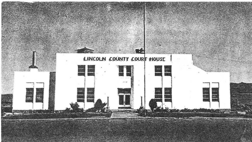
Fig. 7d Lincoln County Court House Pioche, Nevada
